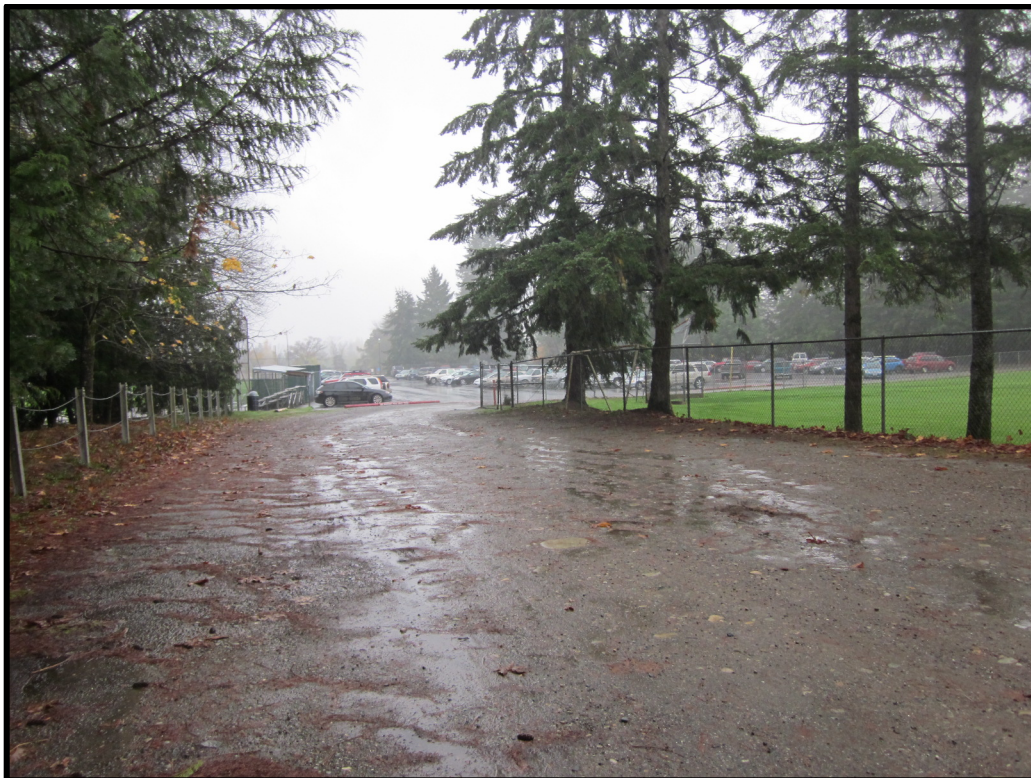
Figure 12. Overview of typical driveway and parking conditions in central part of campus; view is to the south.
