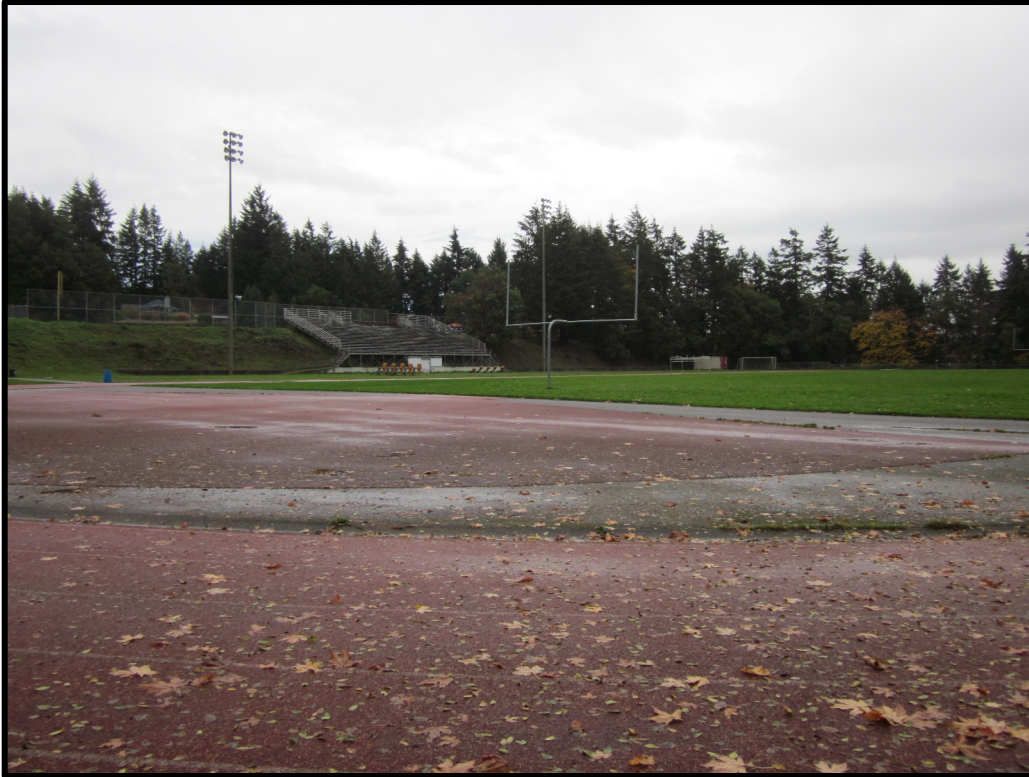
Figure 9. Existing High School football field conditions, with cut slope at left; view is to the northeast.
